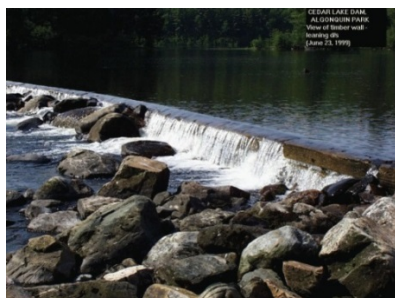
Figure A1.2. Two Algonquin Provincial Park dams — a small dam on Cedar Lake that has with a timber weir about 30 cm tall (above left; photo taken in 1999) and a large 2.5 m high concrete stop log dam on Joe Lake (above right).
