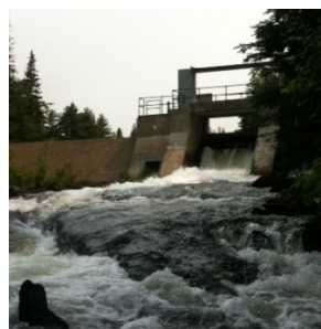
Figure A1.2. Two Algonquin Provincial Park dams — a small dam on Cedar Lake that has with a timber weir about 30 cm tall (above left; photo taken in 1999) and a large 2.5 m high concrete stop log dam on Joe Lake (above right).
